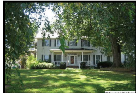
Project Rescue main house
